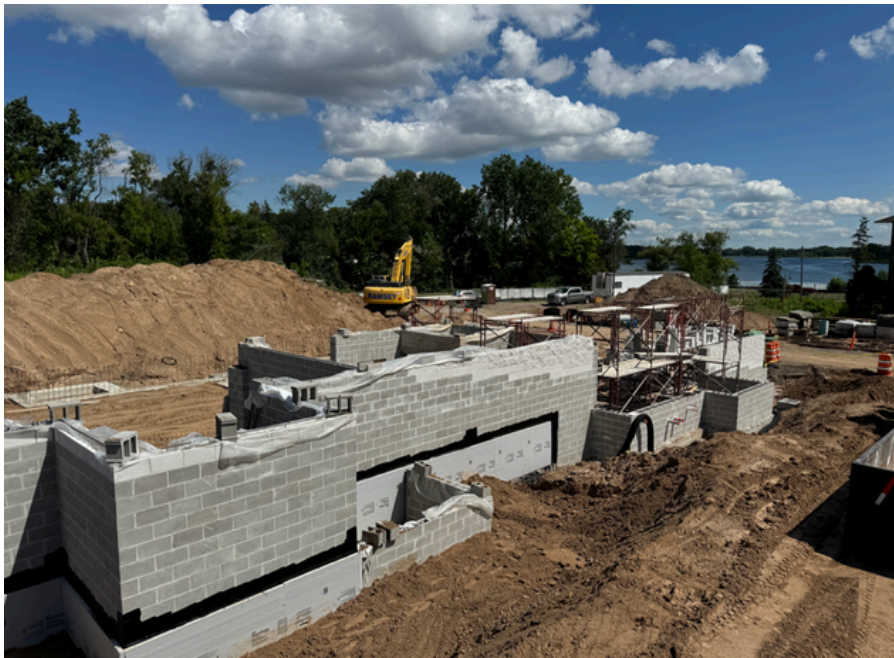
View of Lake Phalen from 1st floor facing south
